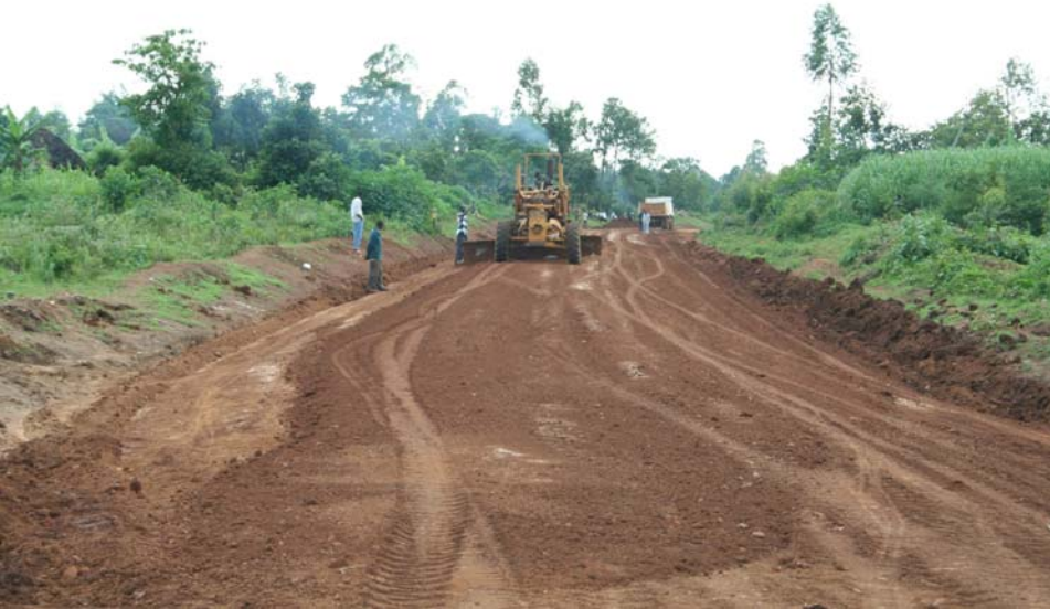
A section of Bokoli-Kimilili Road gravelling project.
