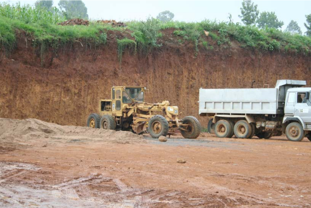
Broken down plant and equipment at one of the road project sites
