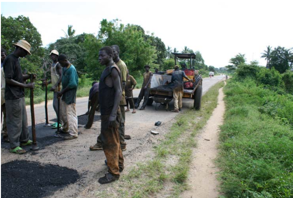
Resealing unit with minimal equipment for pothole patching
