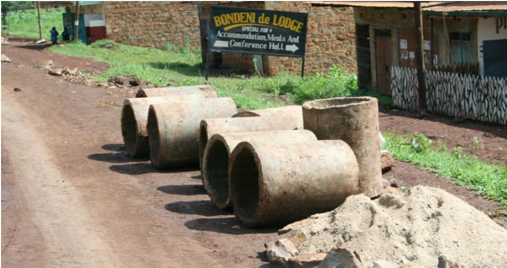
Culverts assembled for laying
