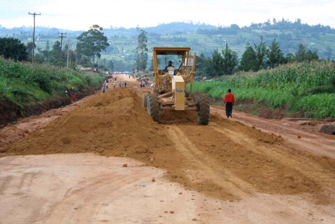
A section of Keroka Nyanguso Road. Work in progress
