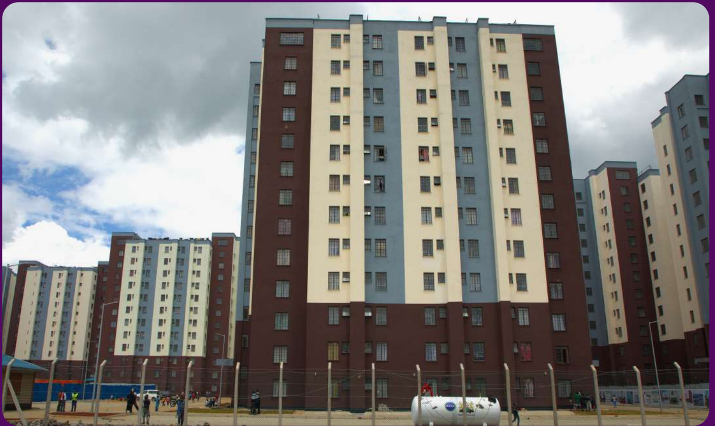
Transforming recovered assets into public value: EACC successfully recovered a 56-acre parcel of land along Mombasa Road in Nairobi's Industrial Area, valued at USD 38 million. Originally owned by the Meteorological Department, the land is now utilized for the development of 15,000 affordable housing units.
